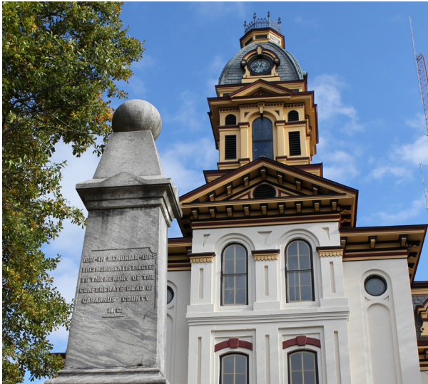
Cabarrus County Courthouse, Concord, North Carolina
